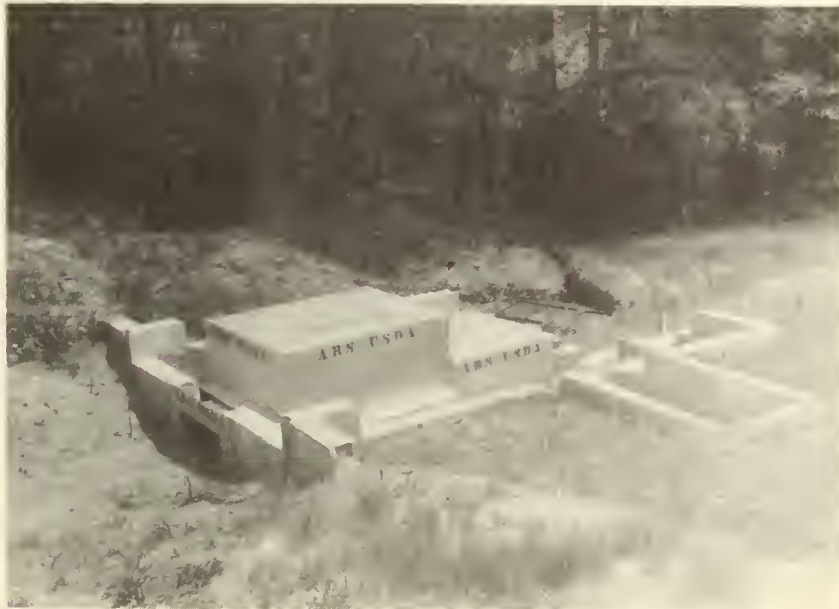
Figure 3.--An overall view of a soil and water measuring device in the lower end of the plot ditch. The black, covered, 54-cubic-foot storage tank is in the background where the 0.5-percent sample is collected.
